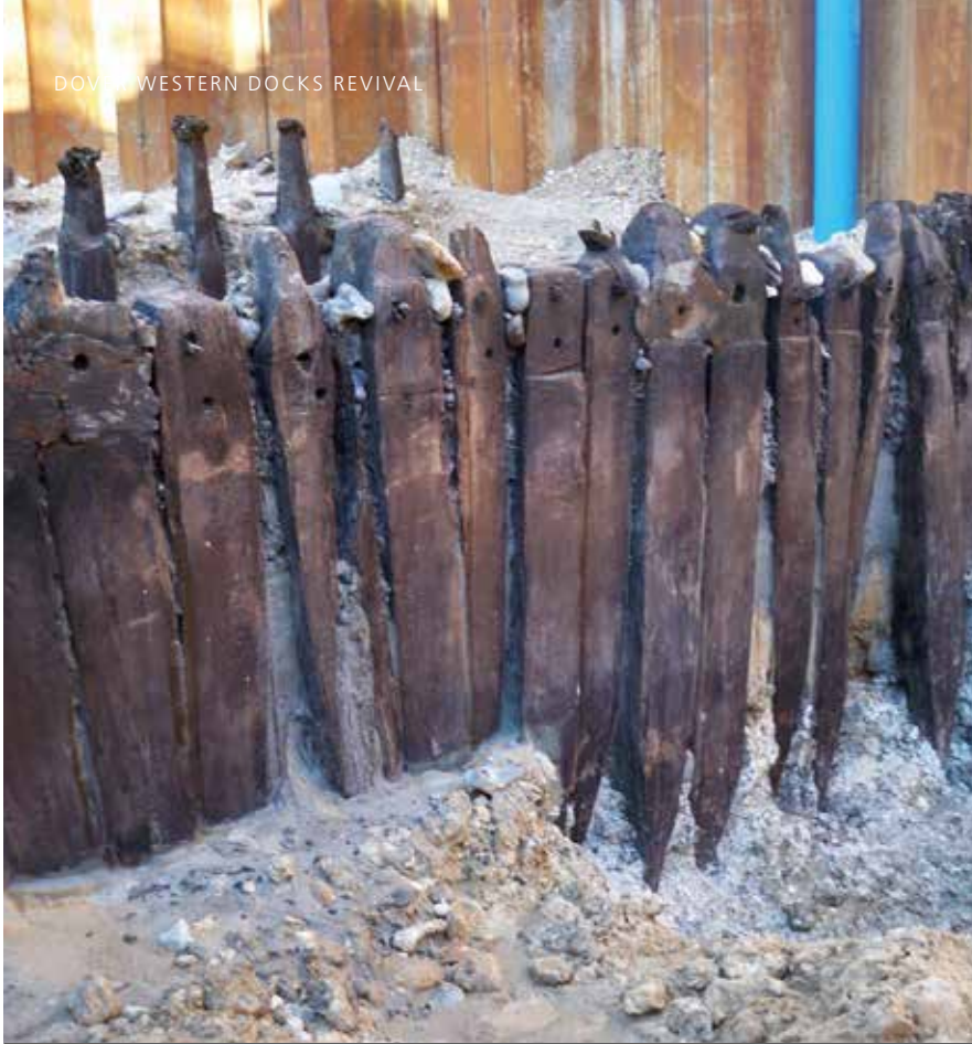
Arrangement of exposed timber wall. c.1661.
