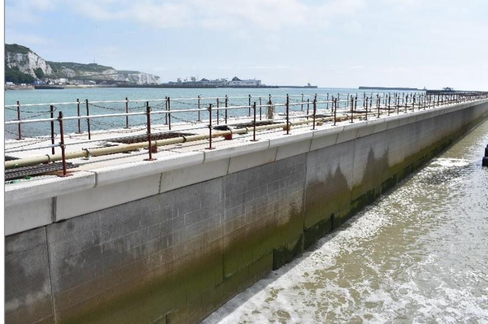
Reclaimed marine timbers have been sourced from the reclamation area and will be fixed vertically to the face of the new Marina Pier to add to the mix of different surfaces on which organisms can grow. These measures are designed to be maintenance free once constructed, allowing algae to inhabit the area naturally, which would occur at a slower rate on a smooth surface.
