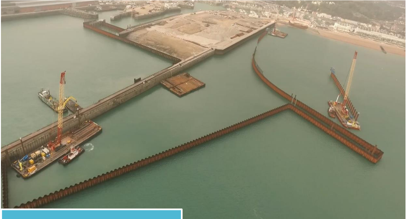
Piling works creating new Port footprint
