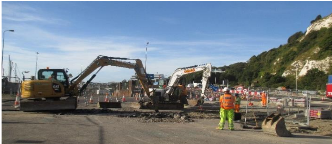
Excavation work continues on Union Street in order to build new kerb lines
